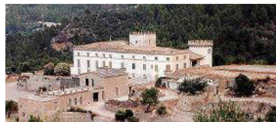
Before, above, and after, top, .....the hotel starts to take shape. PHOTOS: JOAN LLADO.
