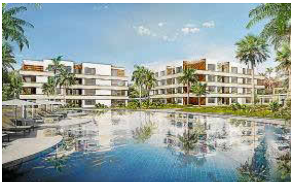
The new Kimpton hotel which is under construction in Santa Ponsa PHOTO: GRAS REYNES ARCHITECTURE STUDIO/WEBSITE
